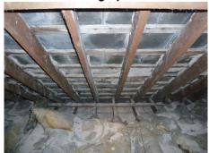
View of underside of the main roof where the lime torching has perished
