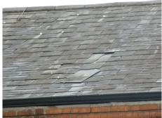
View of slipped and defective slate coverings to the main roof
