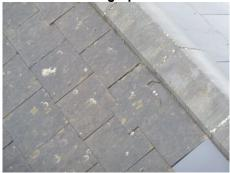
View of what appears to be asbestos based roof tiles over the rear extension
