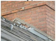
View of cracked and defective slate flashings to the main chimneystack
