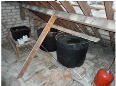
View of exposed and un-insulated cold water storage and expansion tanks
