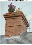
View of foliage growth, perished pointing and spalled brickwork to the rear chimneystack
