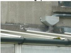
View of inadequate temporary flashings to the conservatory roof
