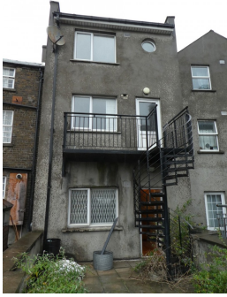
General view of the rear elevation
