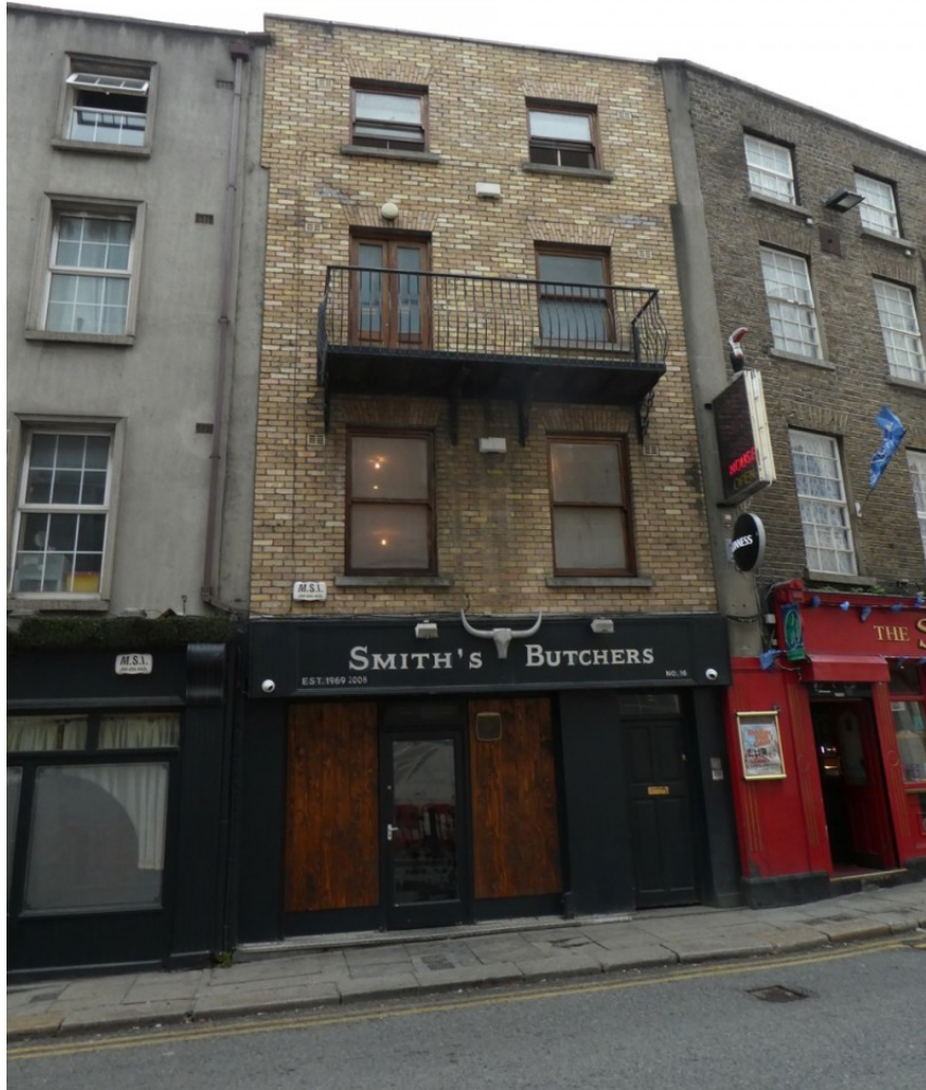
View of the Front Elevation
